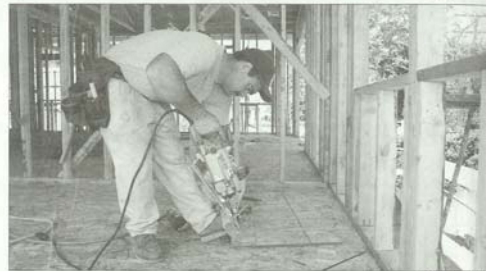
Structure: Work is underway on three predesigned houses in Brentwood.
